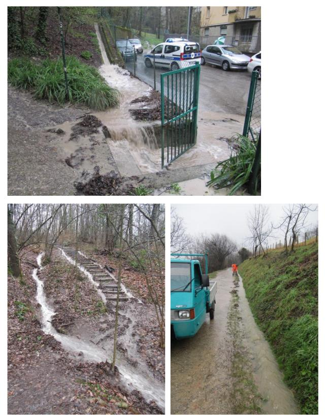
The more and more frequent and intense rains concentrated in a short time cause significant damage in the network of paths and in the regulation of surface water in parks and gardens. Some examples in the Park of Villa Ghigi in Bologna: one of the secondary entrances (upper picture) and two sections of the path network (lower pictures).
